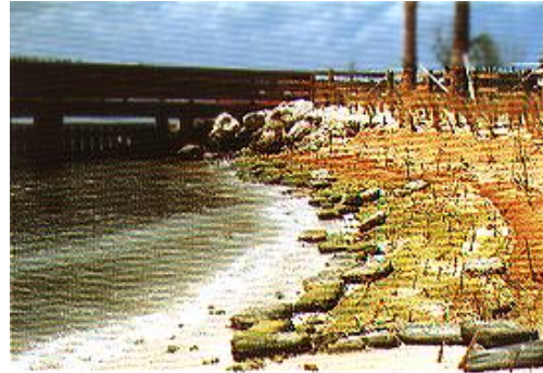
GEOCOIR®/DeKoWe® 700 being used in a vegetated geogrid and blanket application to protect a sand embankment from tidal and pleasure boat wave action.
