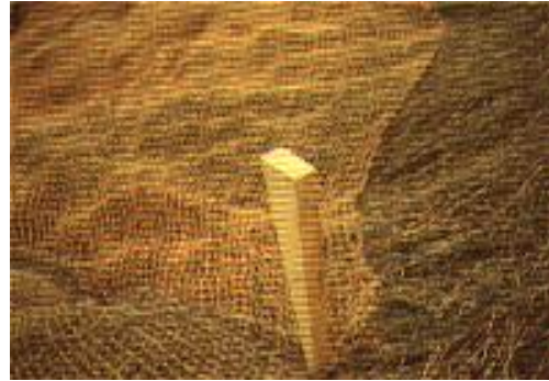
Secured by using wooden stakes as pictured here.
